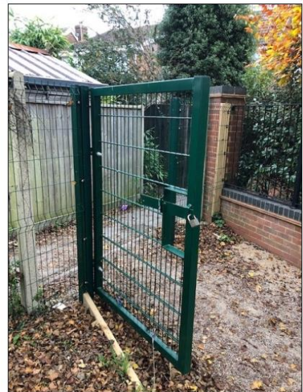
New reinstated pedestrian gate to improve access on to adjacent paths
