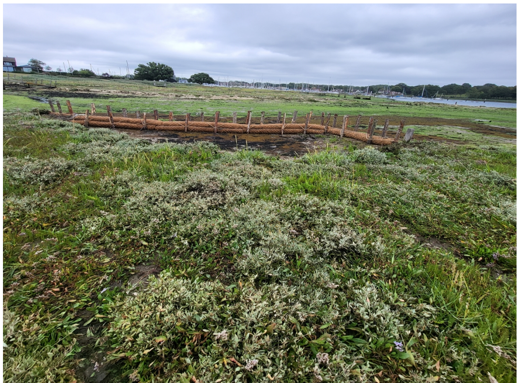
Newly installed sediment retention barriers to encourage sediment accretion and plant colonisation to drive saltmarsh habitat recovery, Hamble Estuary (photos courtesy of Solent Seascape Project).
