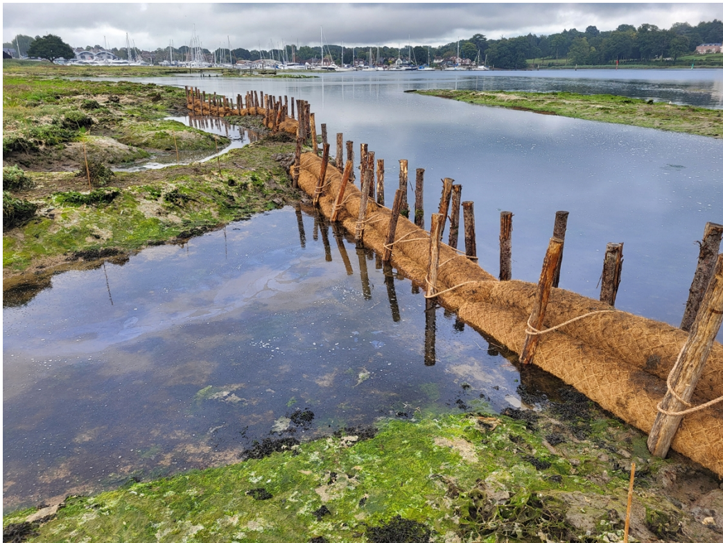
Newly installed sediment retention barriers to encourage sediment accretion and plant colonisation to drive saltmarsh habitat recovery, Hamble Estuary (photos courtesy of Solent Seascape Project).
