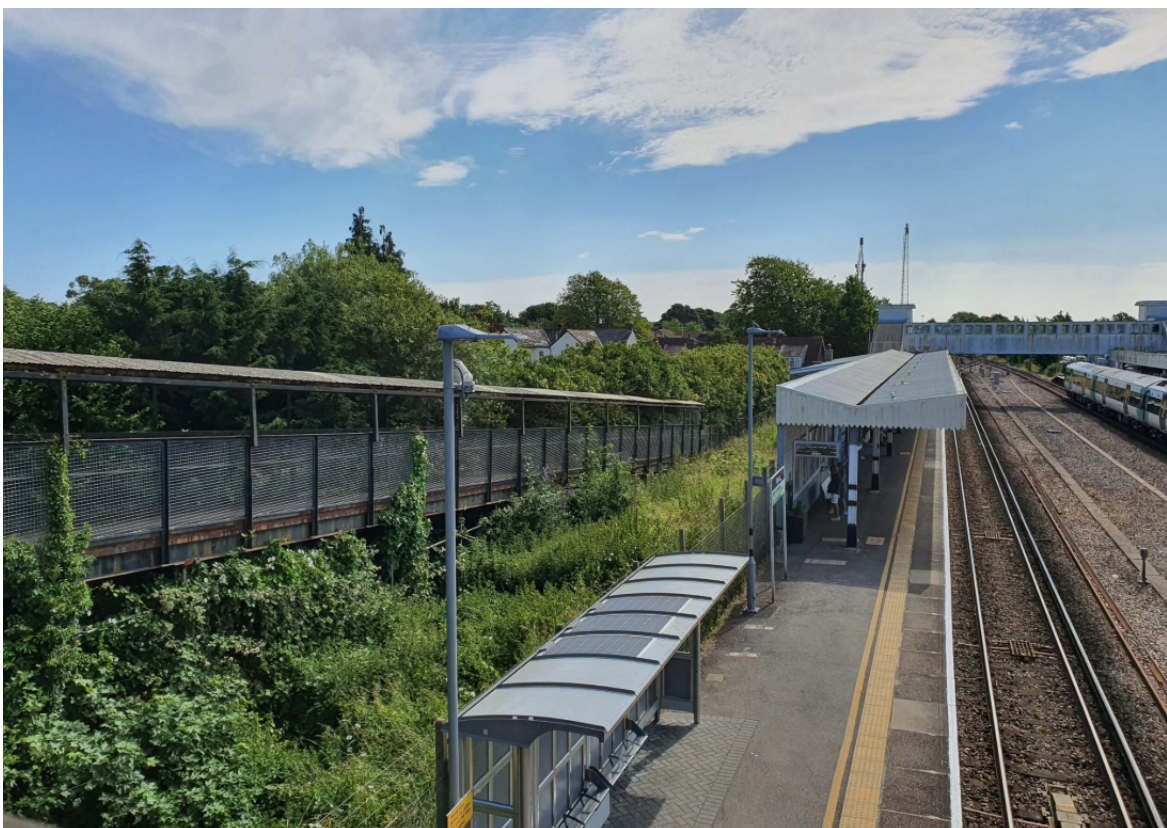
North east ramp – now closed
