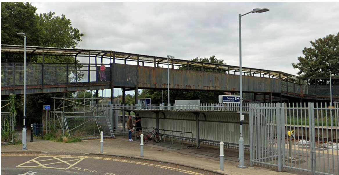
East elevation of Havant Footbridge.
