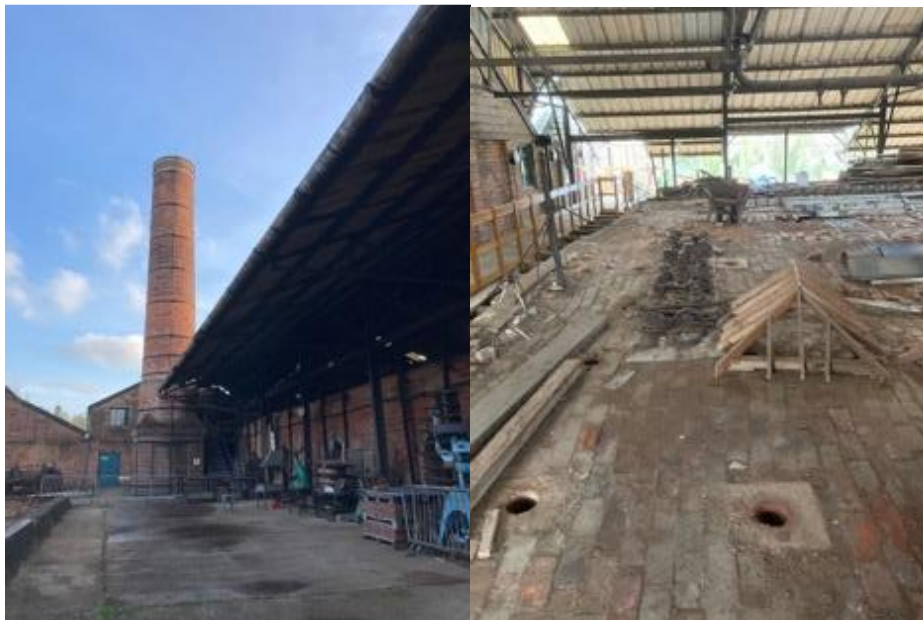
The Kiln (to the right of the photo) and the kiln roof showing fuel feeds
