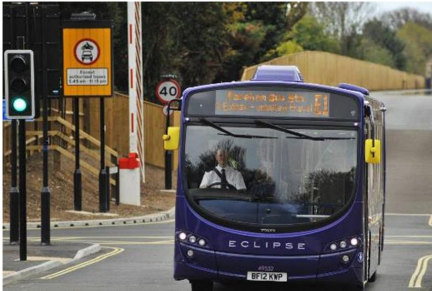
Figure 12 – The Fareham-Gosport BRT busway
