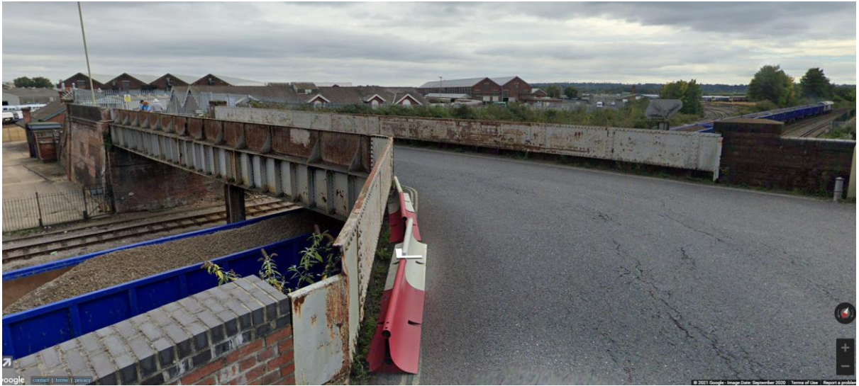
View on top of bridge
