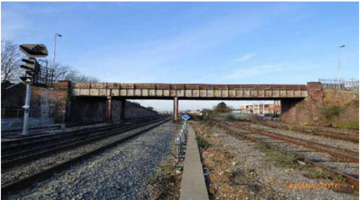
Elevation of bridge from track level
