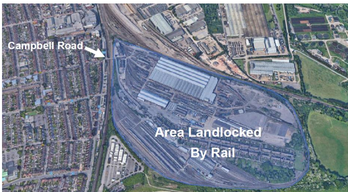
Campbell Road bridge location and area served.
