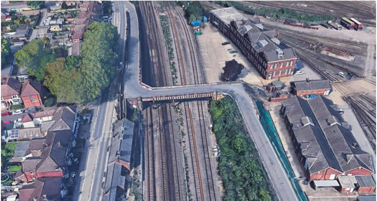
Aerial view of Campbell Road bridge over the Bournemouth Main Line (left) and sidings (right).
